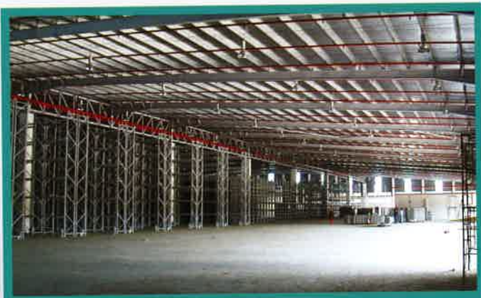
BMW DISTRIBUTION CENTRE
