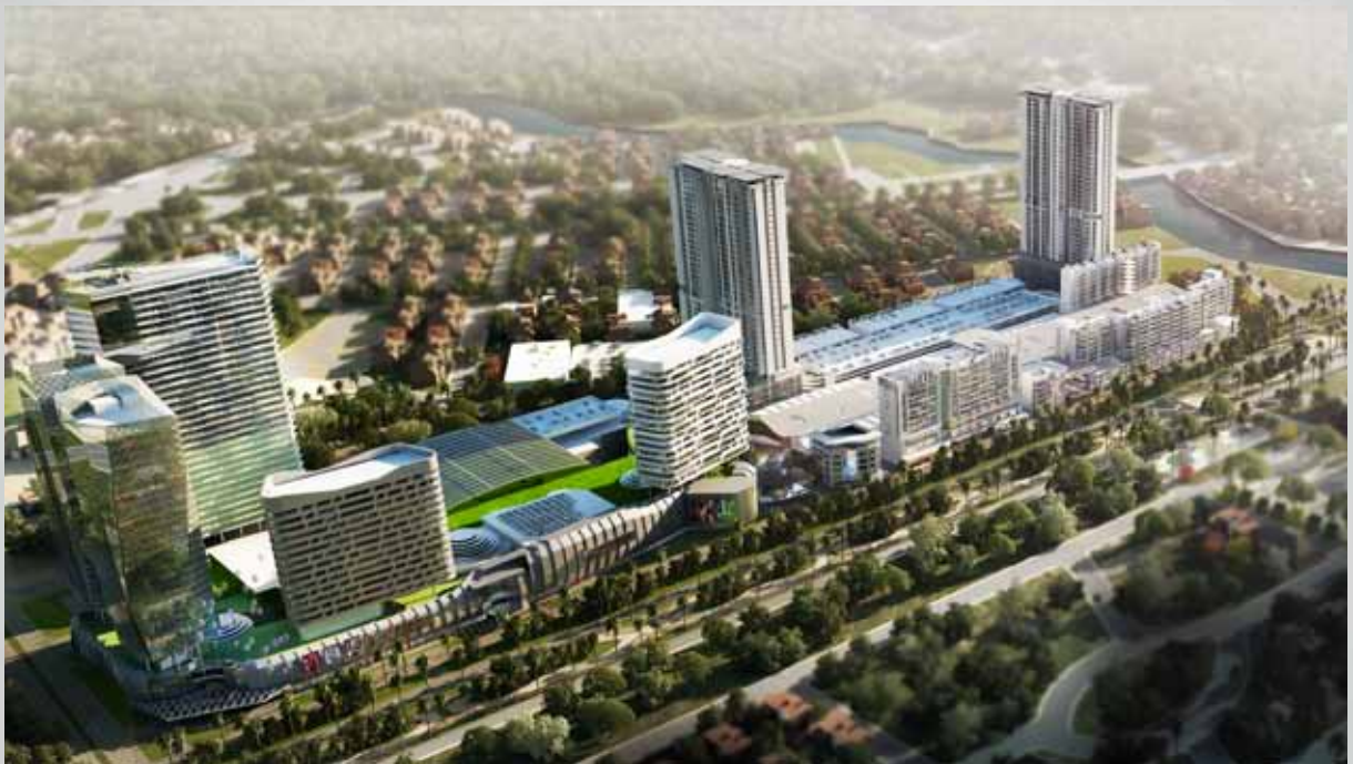
Aerial View, Bintulu Paragon
