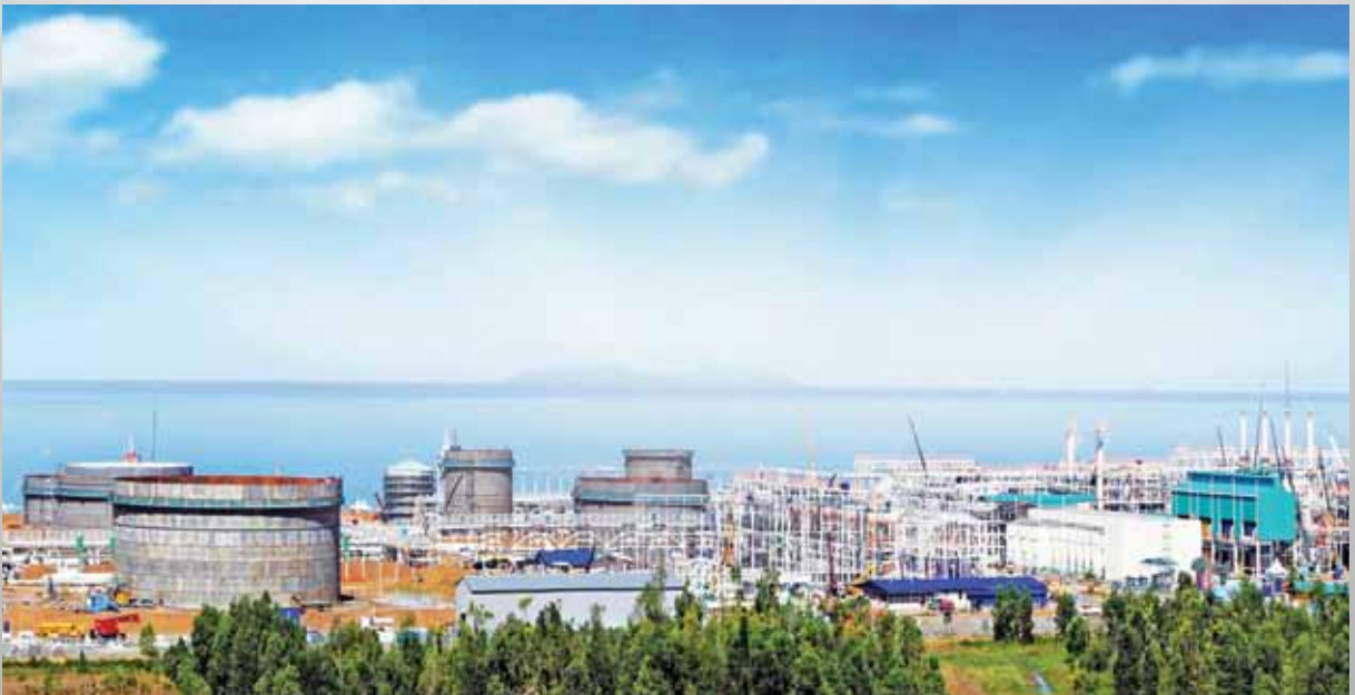
SABAH OIL & GAS TERMINAL (SOGT) PROJECT, SABAH
